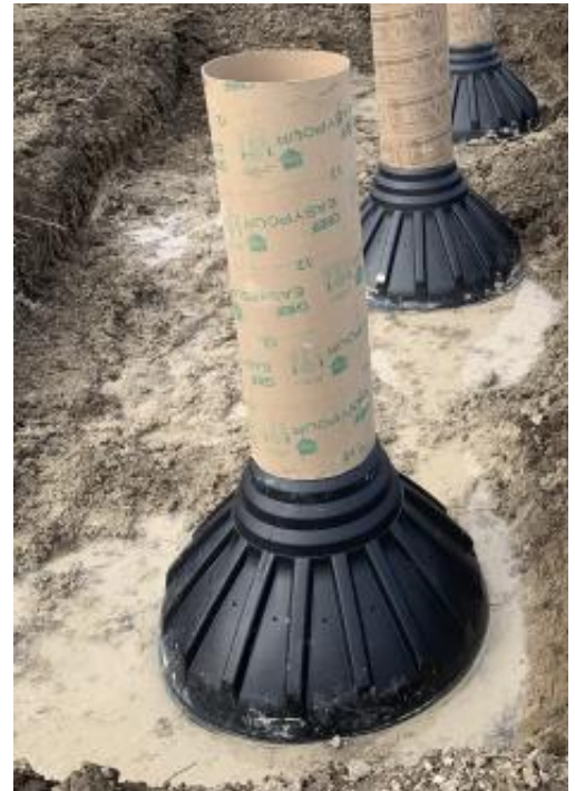
Diagram 3: Pre-molded pier forms
